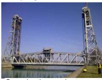
Vertical-lift drawbridges are unique structures. To provide clearance for vessels on waterways, the entire road or rail section is lifted vertically between two towers. Counterweights, equal to the weight of the road section, reduce the amount of mechanical force needed to move the section upward or downward.
